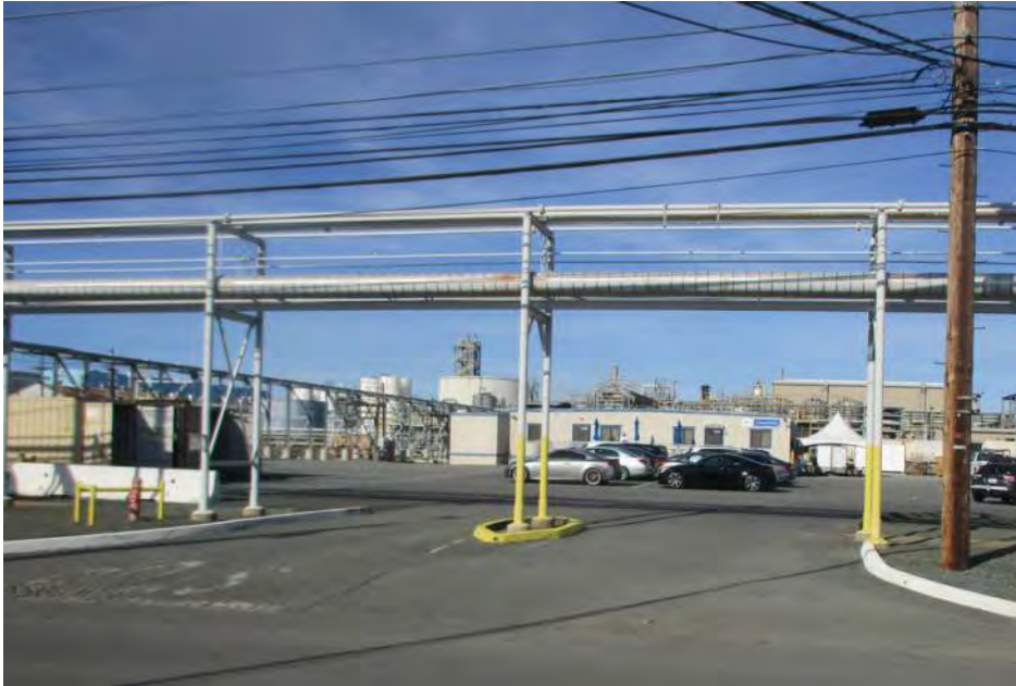
K2 Parking Entrance from E-Street (Elevation of new bridge beam will be near that of upper level of existing pipe rack)
