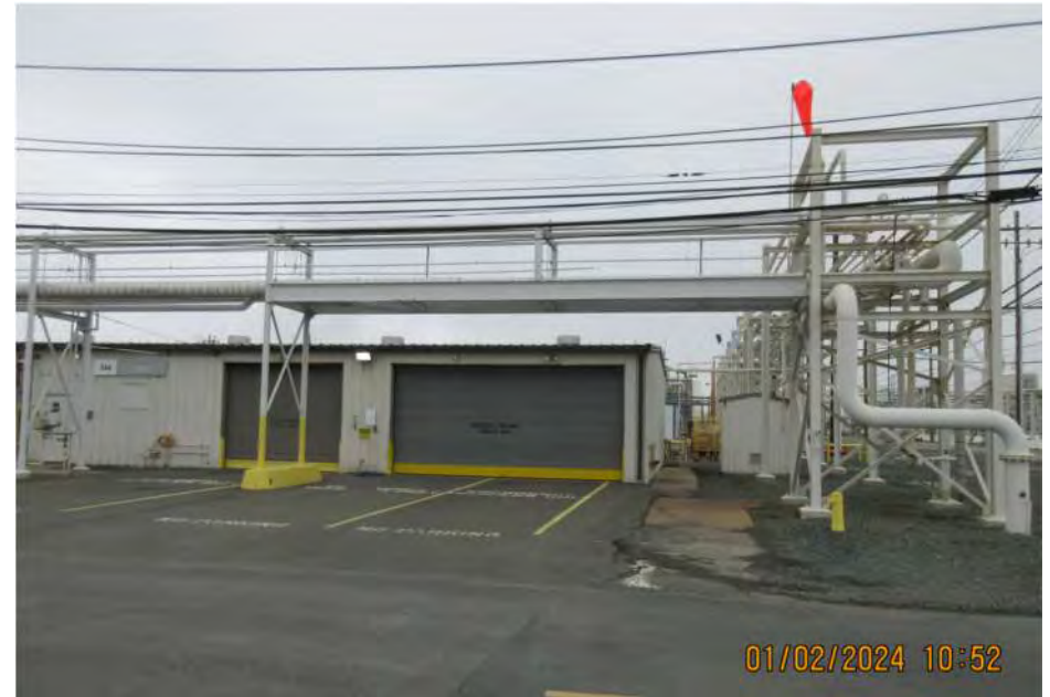
Building 344 Driveways (Elevation of new bridge beam will be near that of upper level of existing pipe rack/bridge)
