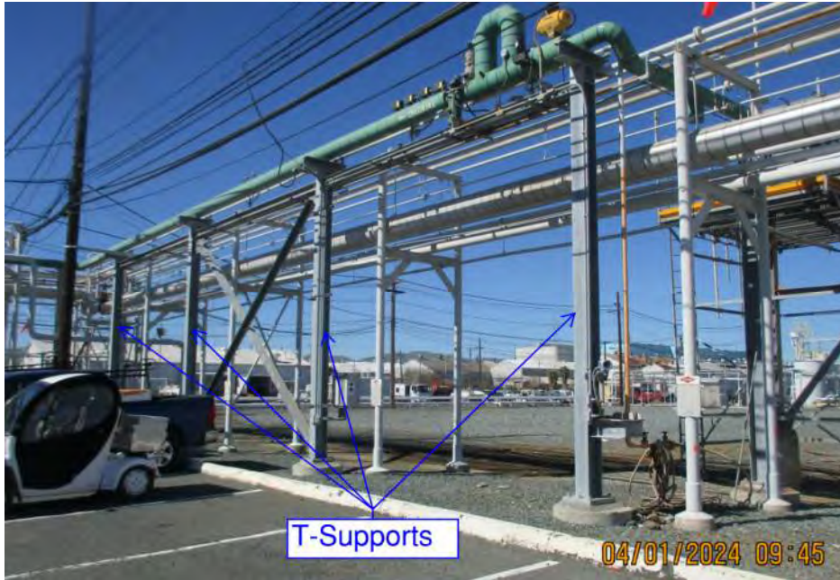
Interconnected Steel T-Supports built in 2011 adjacent to Older Pipe Rack
